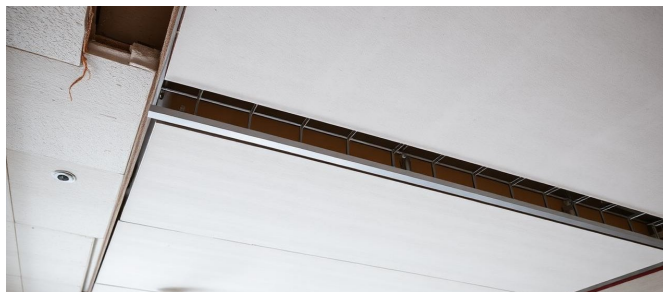
FALSE CEILING FRAMEWORK WORK IN PROGRESS
