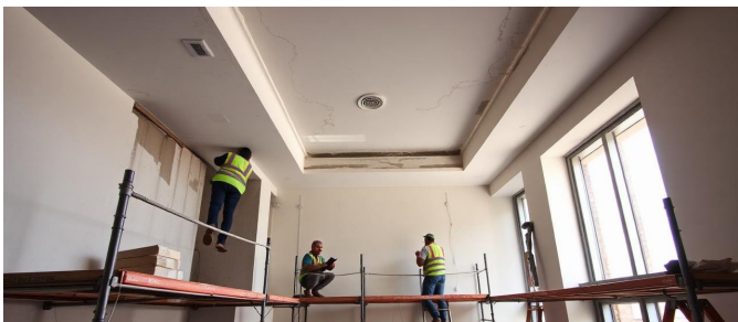
PUTTY & PRIMER STAGE WORK IN PROGRESS
