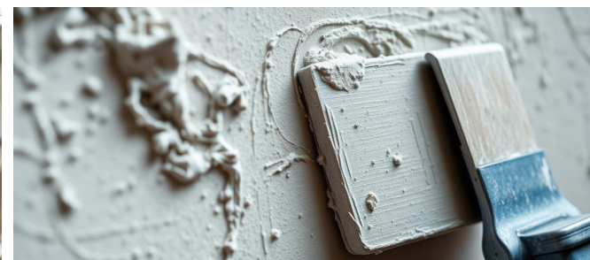
FINISHING DETAIL WORK IN PROGRESS
