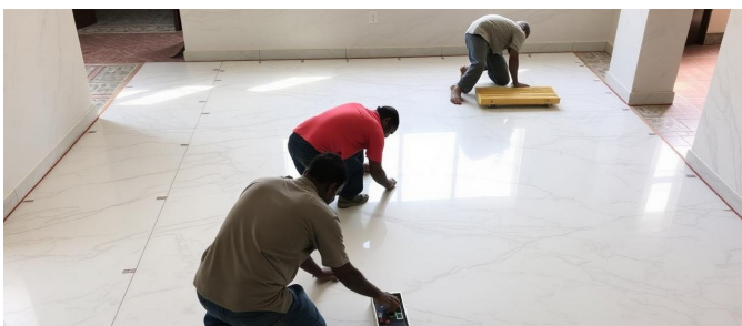
MARBLE FLOORING WORK IN PROGRESS
