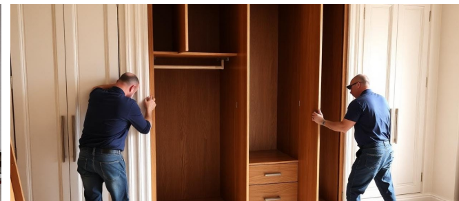
CARPENTRY INSTALL WORK IN PROGRESS
